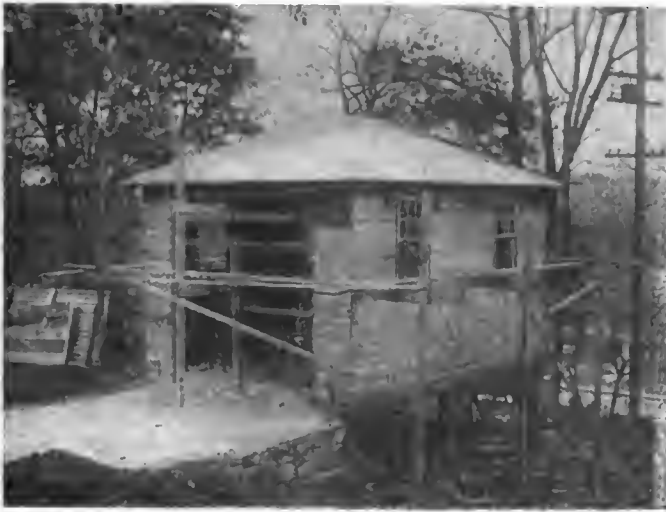
One-Car Frame Garage In Process of Construction
